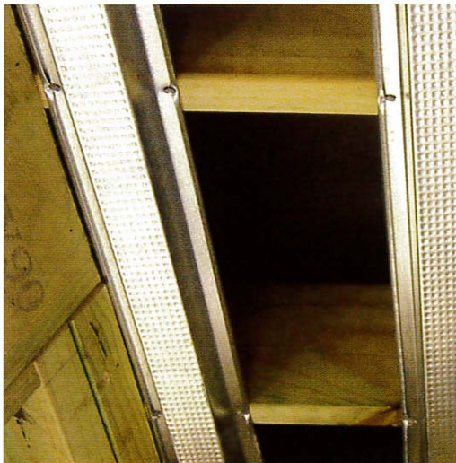
Direct fix to trusses
